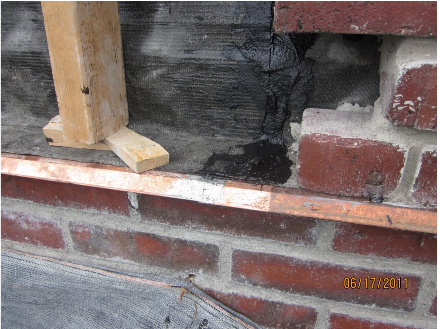
Thru Wall Flashings
