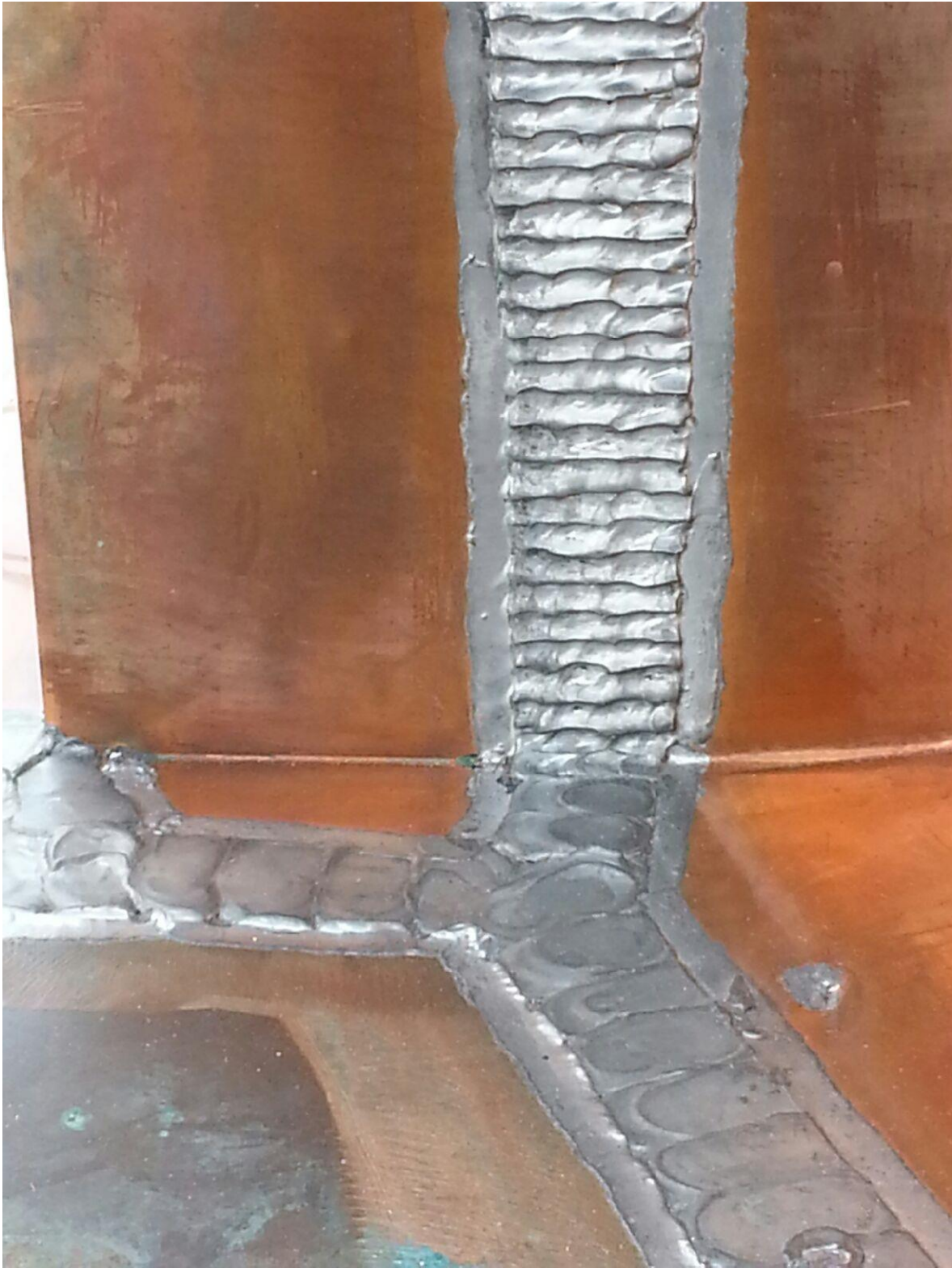
SOLDERING OF COPPER ROOFS
