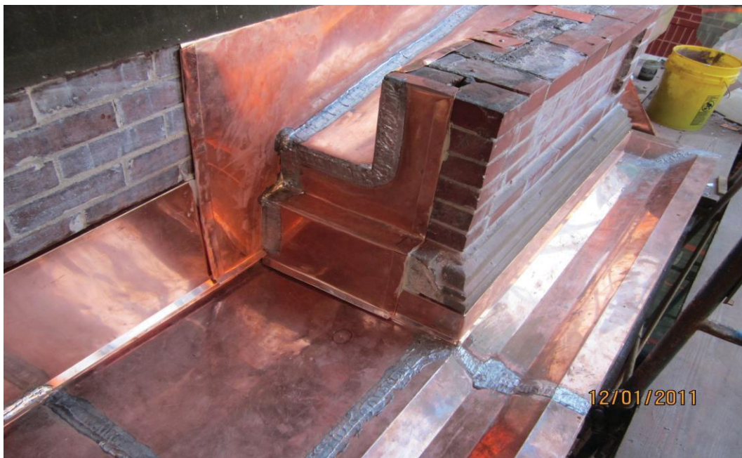
Built in Gutter Systems
