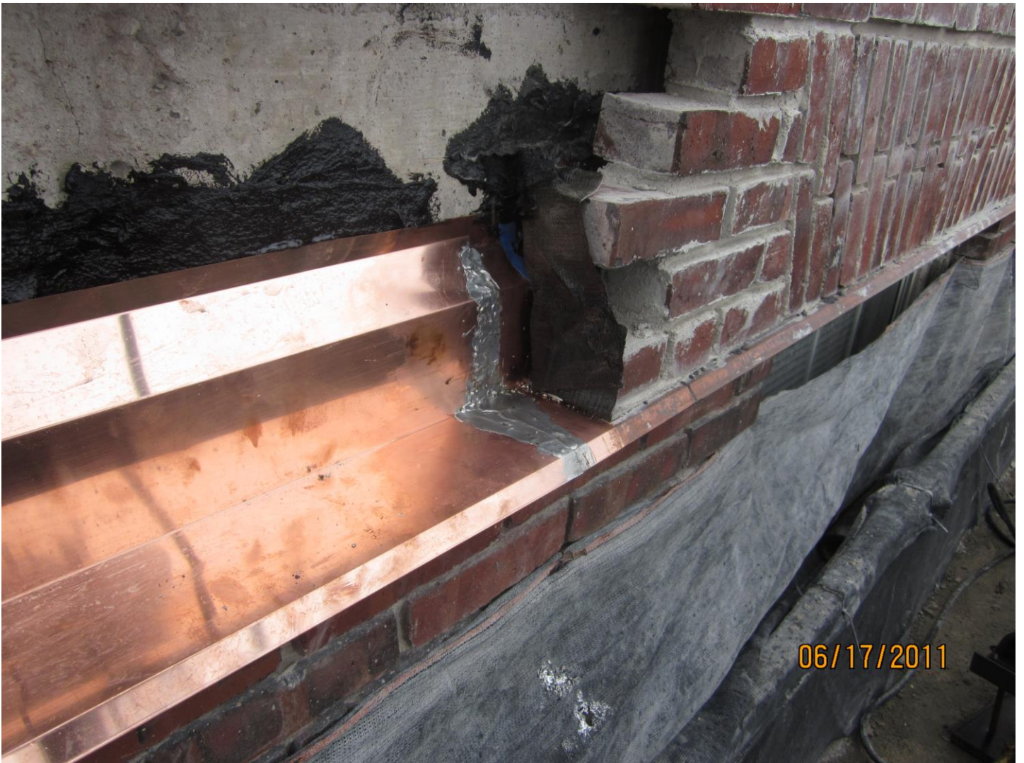
Thru Wall Flashings
