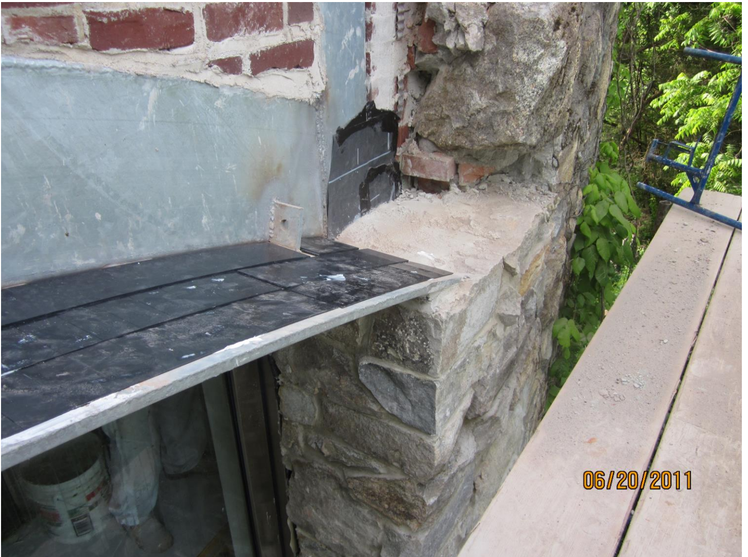
"Before" Thru Wall Flashings
