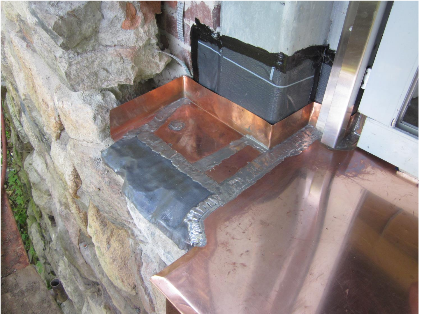
"After" Thru Wall Flashings
