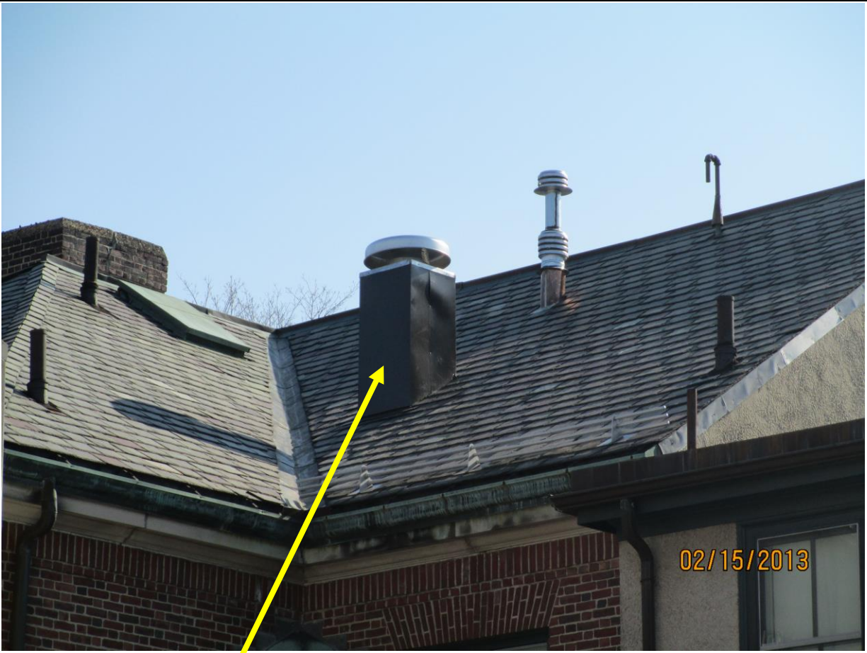
Laundry Chute vent on pitched slate roof
