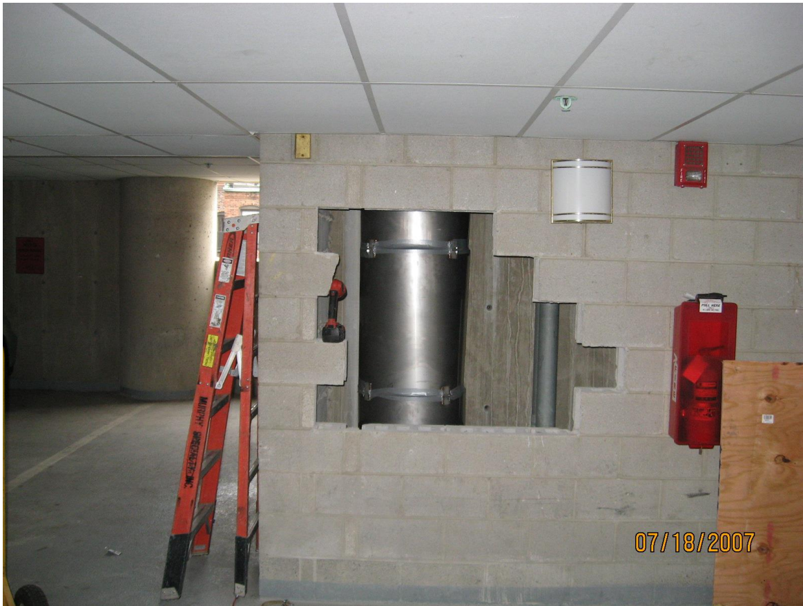
Linen Chute collapsed inside CMU wall
