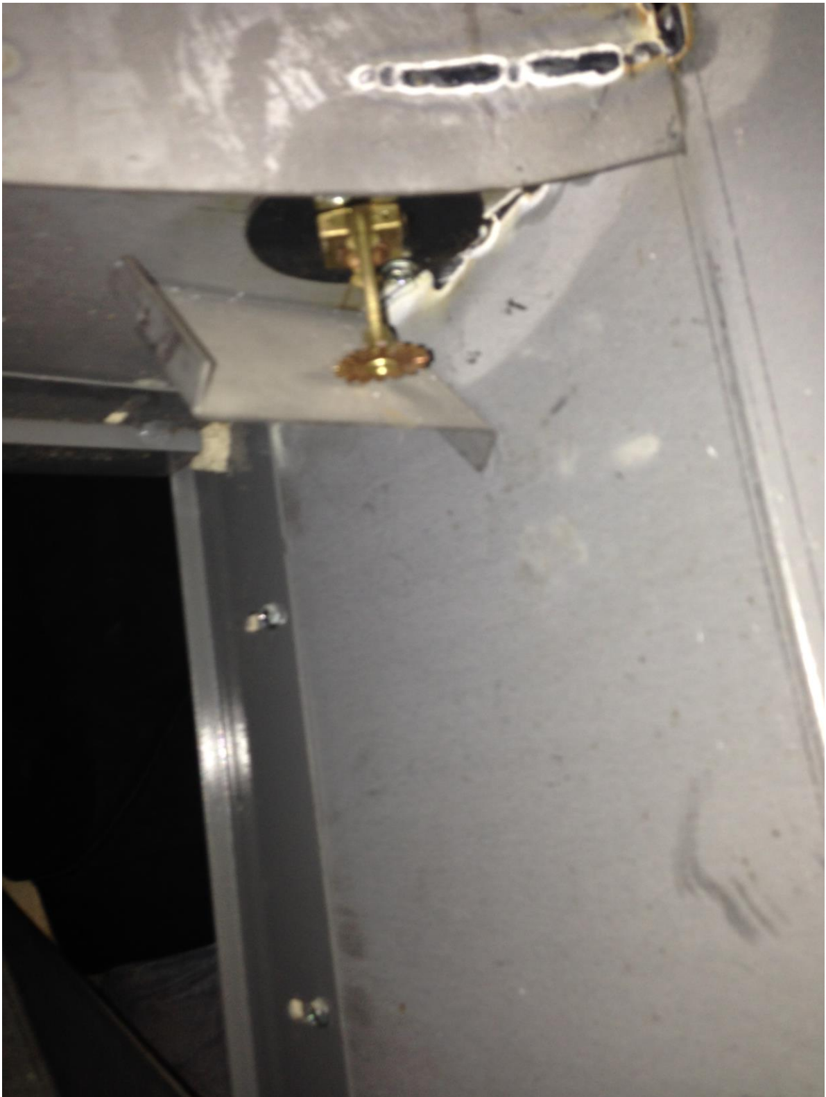
Sprinkler Heads installed in Chute ready for piping
