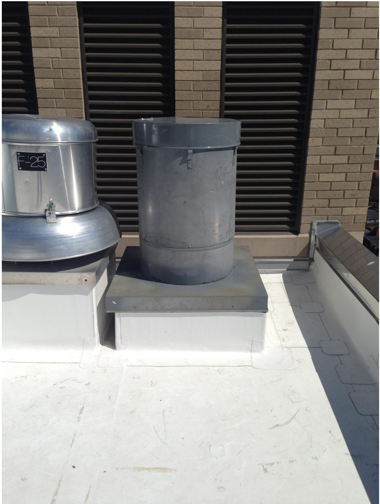
Chute Vent – 4' above roof line
