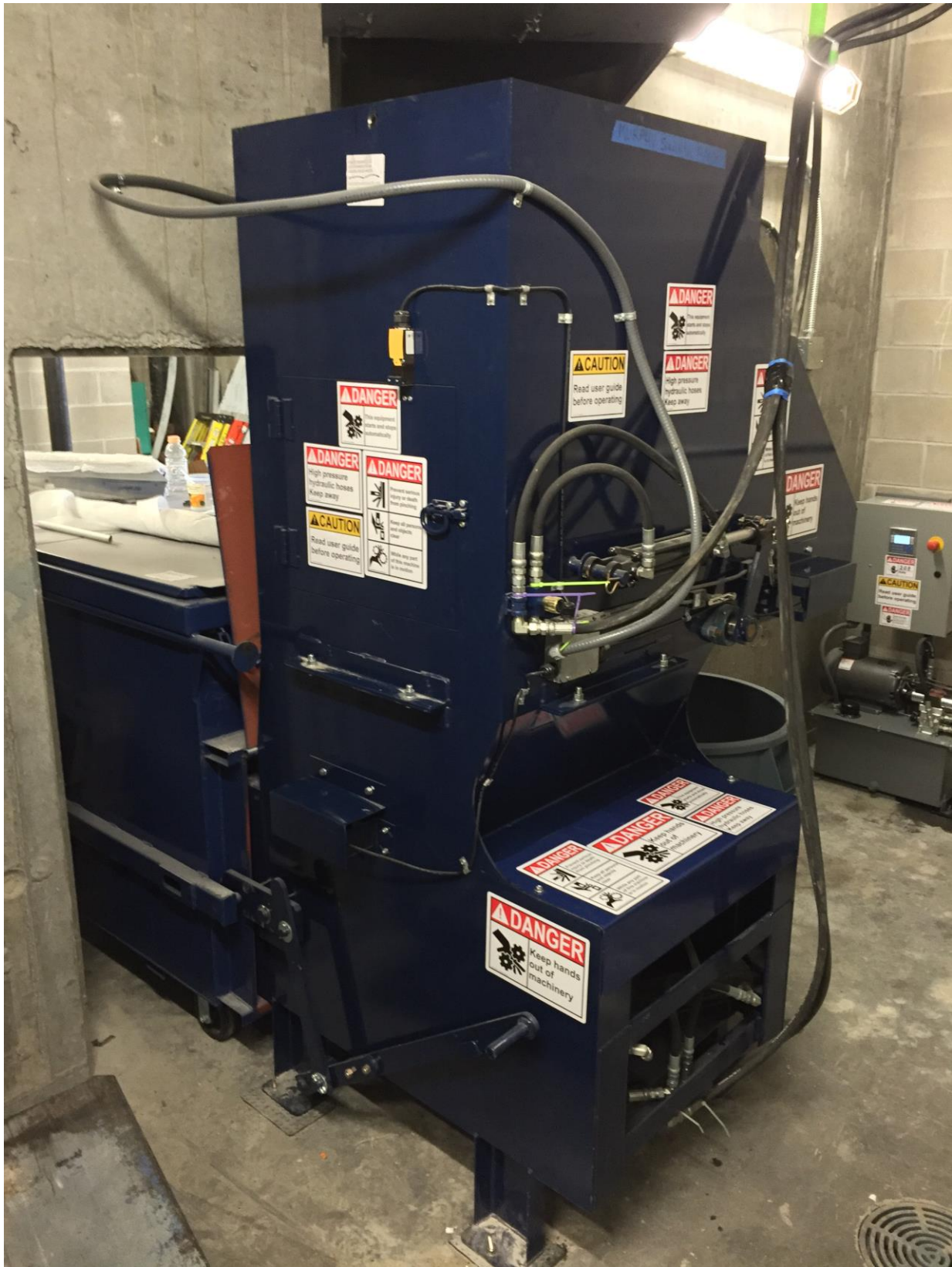
BI-Sort ( Compactor and Recycle System )
