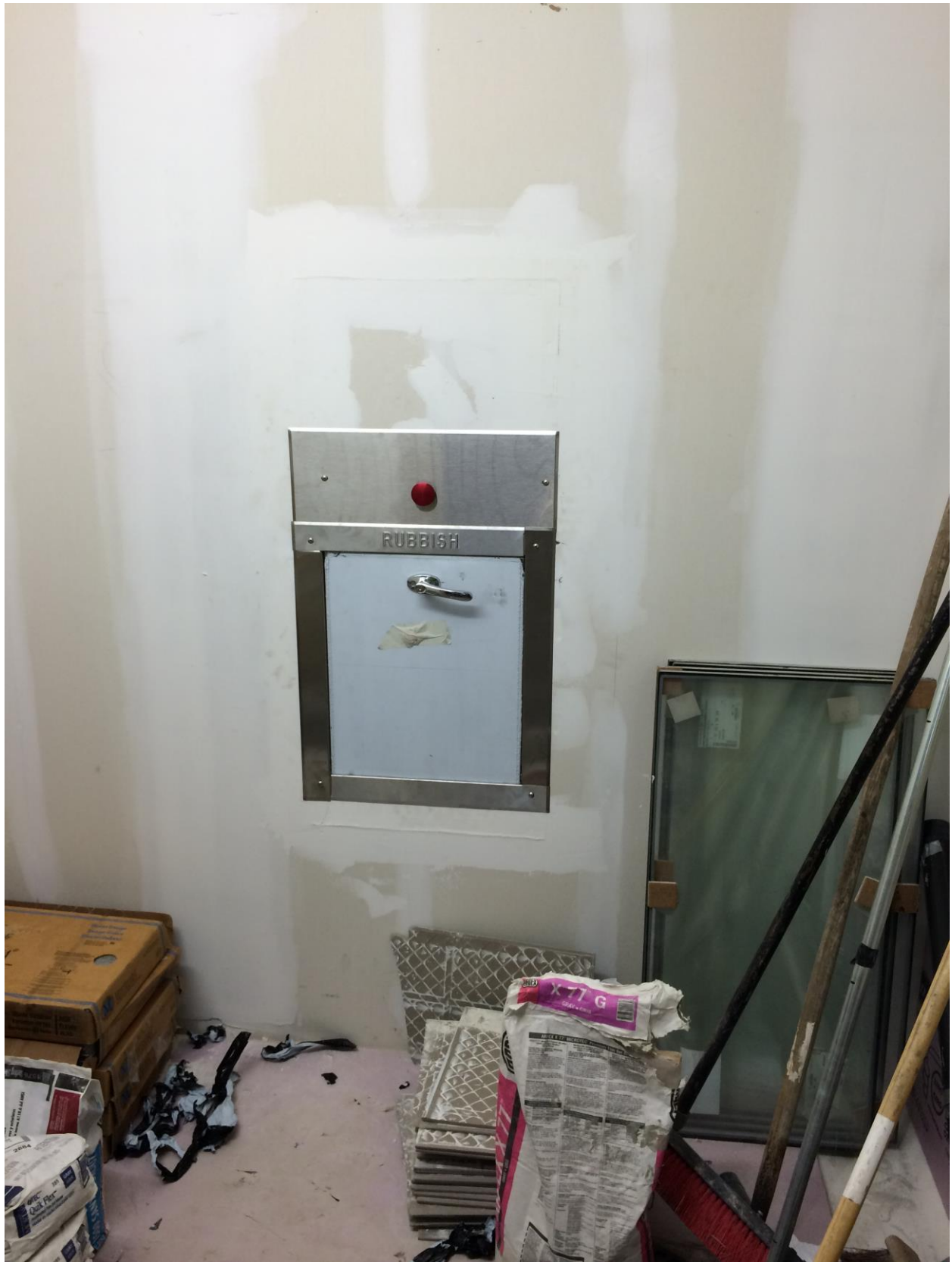
Pneumatically / Palm button operated doors with keyed LEVER handles
