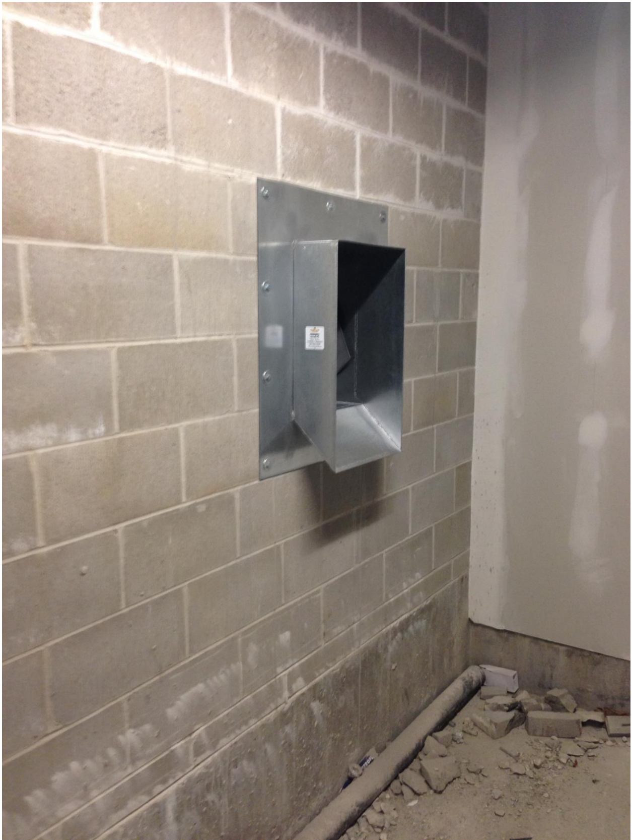
Through Wall - Chute door and sleeve
