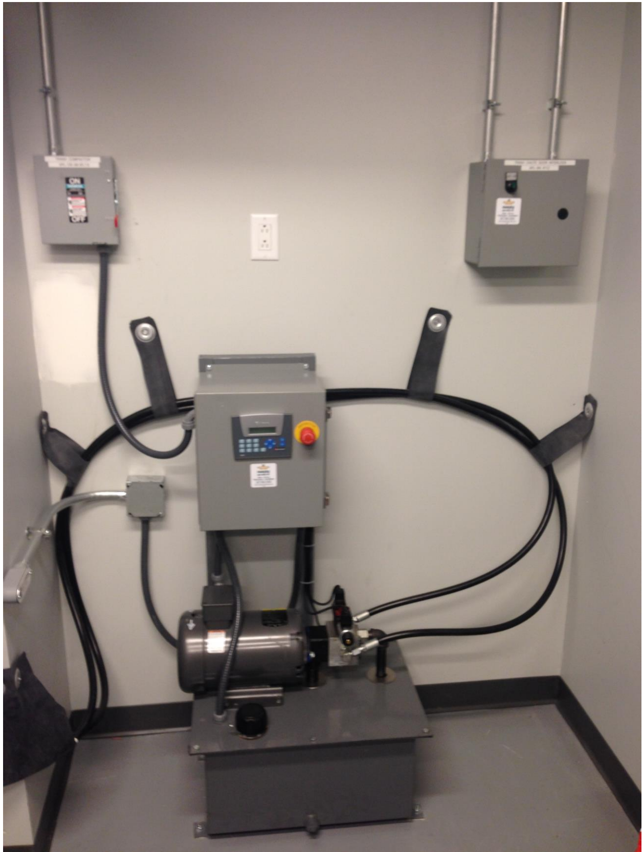
Compactor / Recycle System's hydraulic control panel
