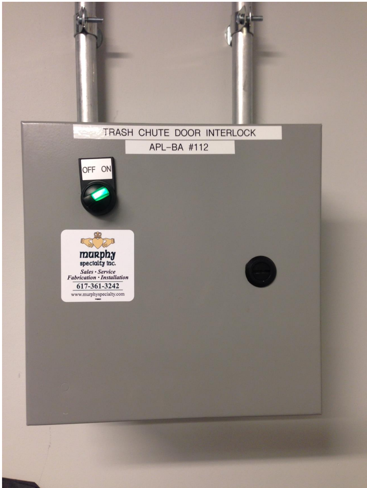
Electrical Interlock Control Panel – Locks out Chute Doors
