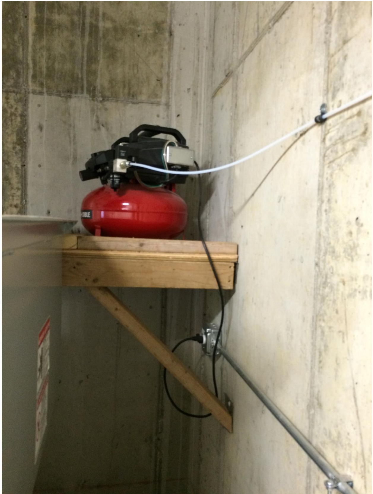
Air compressor used for the door operation
