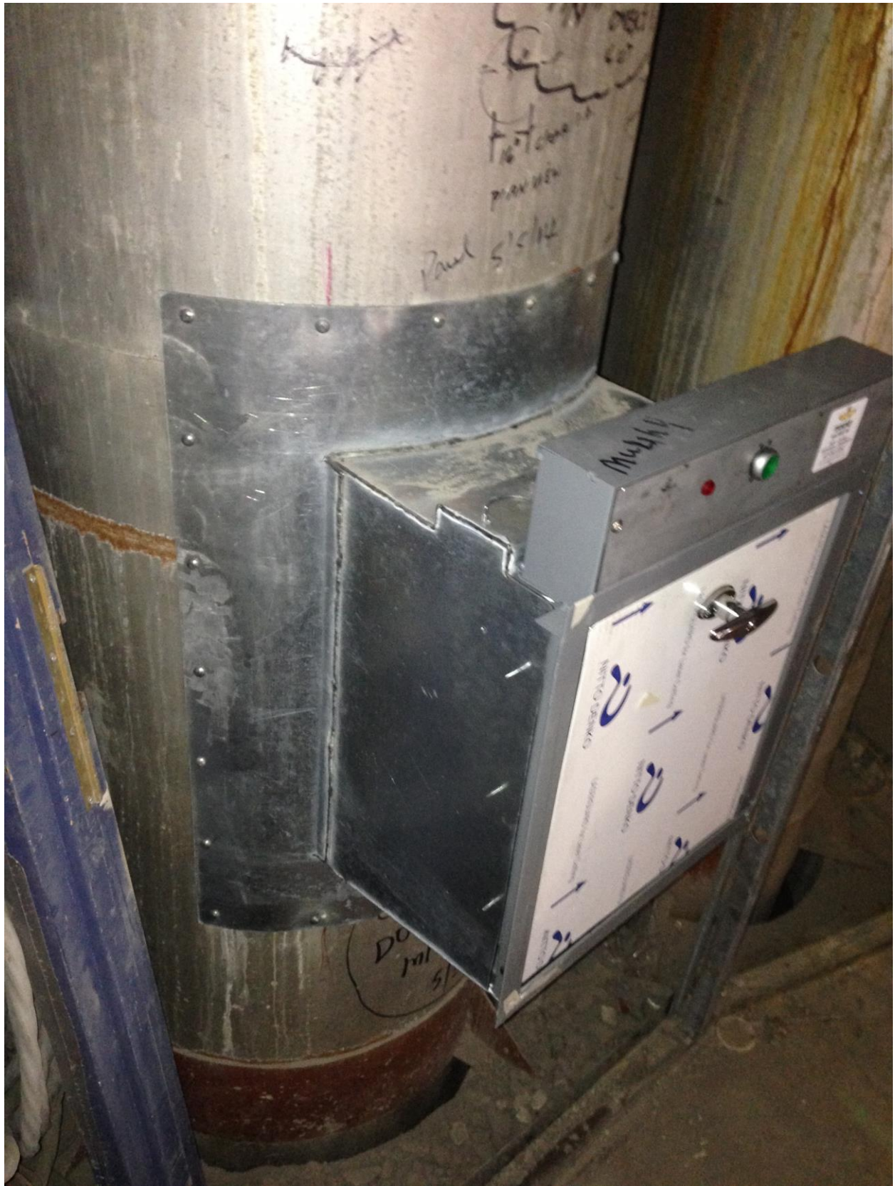
Existing Concrete Incinerator converted with new UL Listed Chute Doors. ( Self Closing and Positive Latching ).
