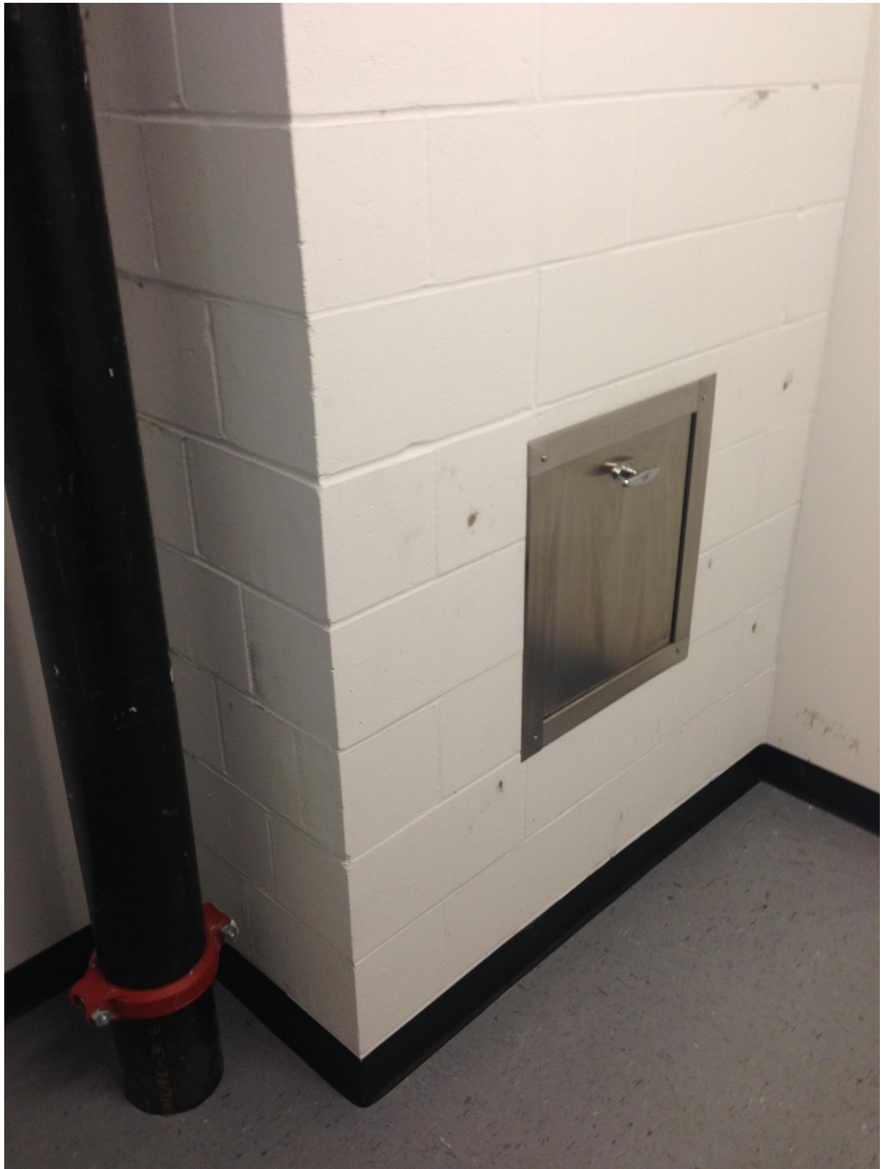
New Chute door flush with CMU wall / shaft. Lockable T Handle
