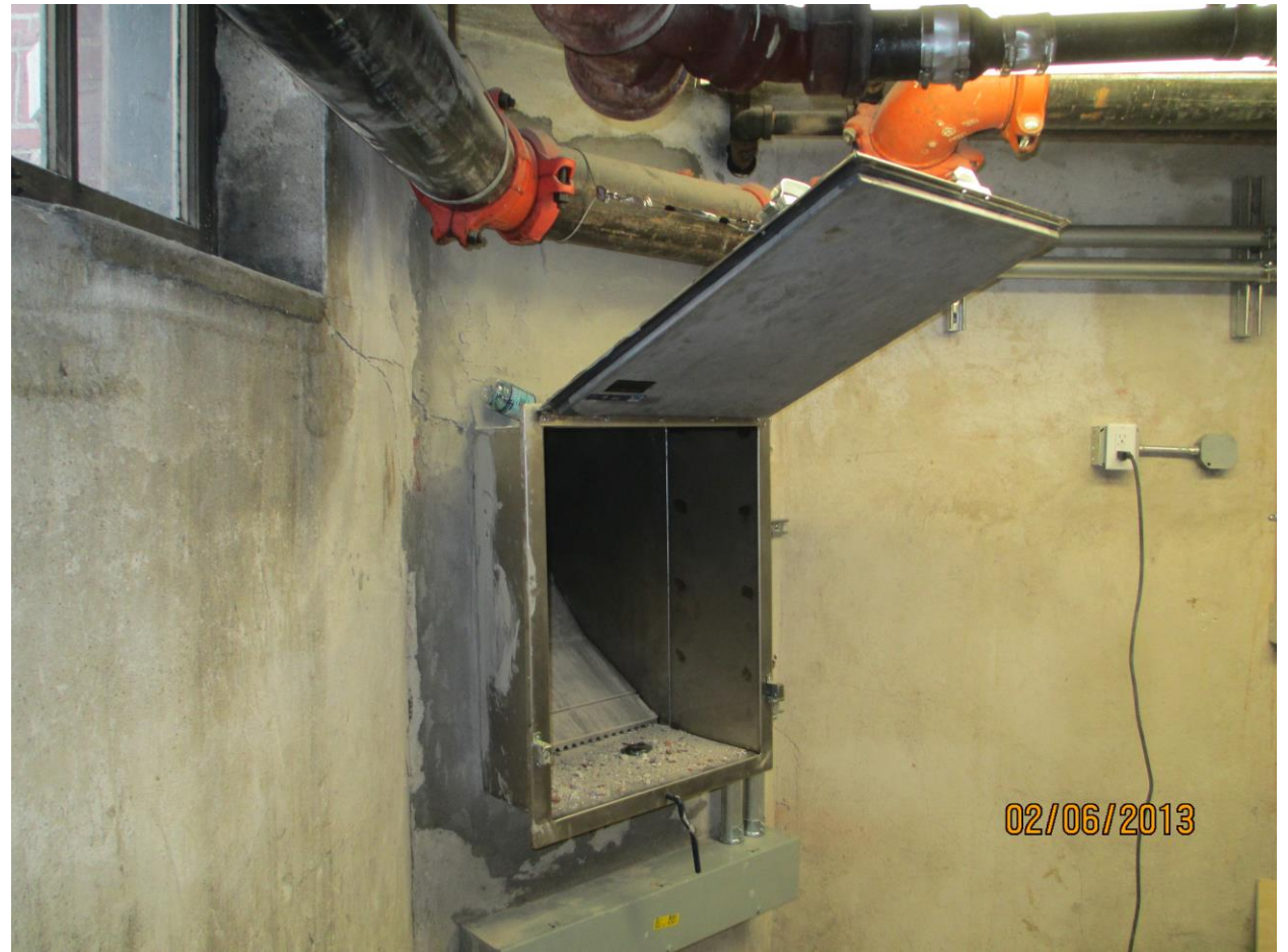
New UL Listed discharge “hopper” style door at bottom of soiled linen chute
