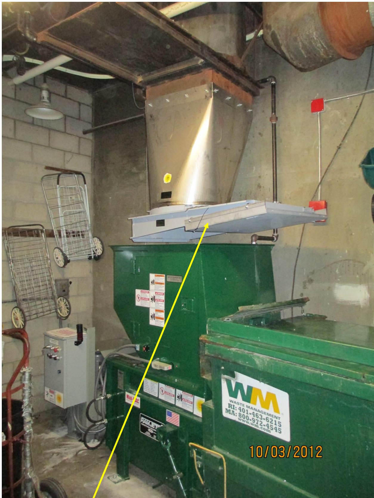
Chute's Discharge Fire door with UL listed Fusible link per NFPA 82
