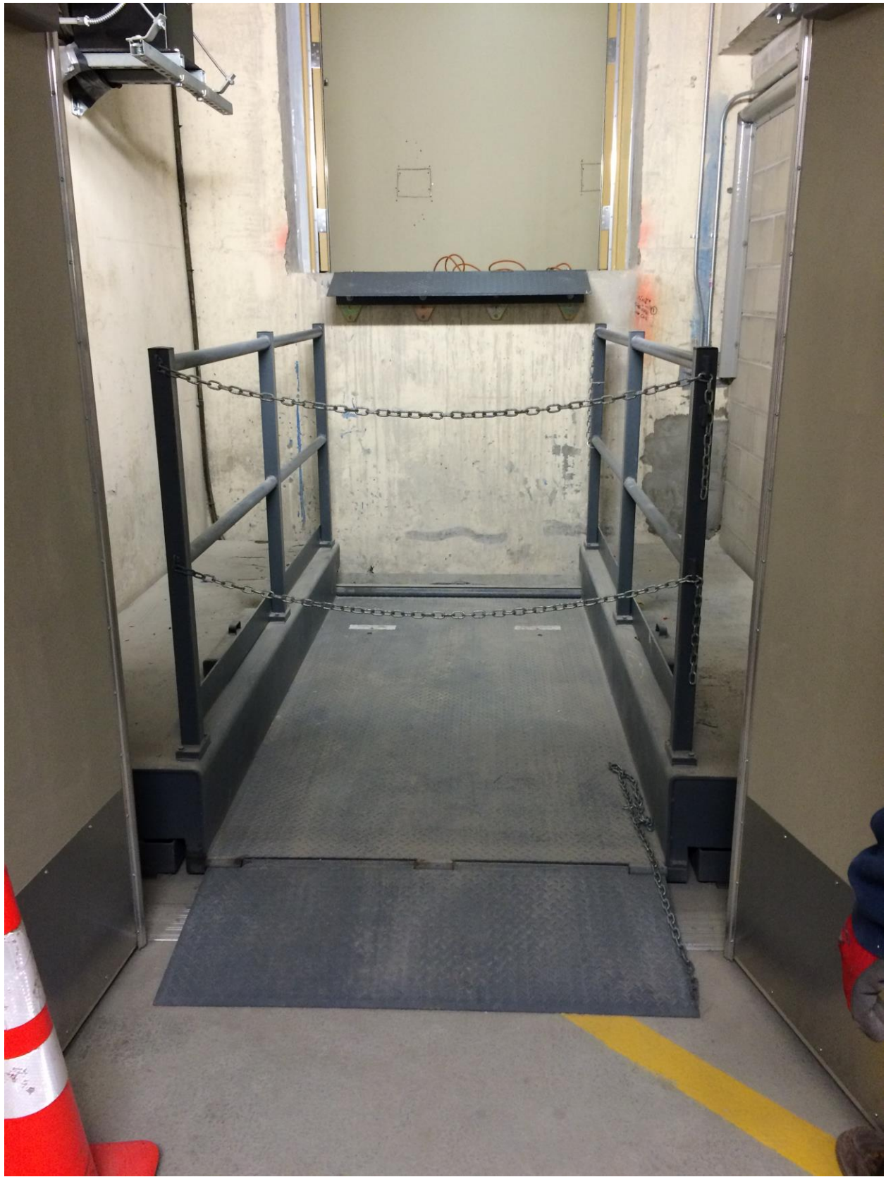
Hydraulic Lift – which raises a Trash Container from ground level to the loading dock.
